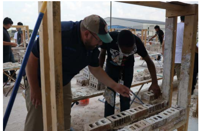
Johnny Johnson with Mr. Blankenship, laying a brick using additional means beyond sight to create a level course
